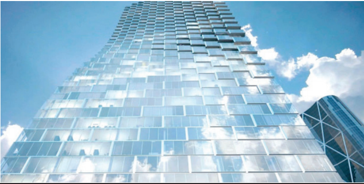
Telus Sky: only 40 per cent of the space is leased in a tower that completes in 2018.
