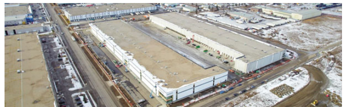
Cool IT leased 114,000 square foot in iPort Starfield Logistics Park Bldg. 4.
